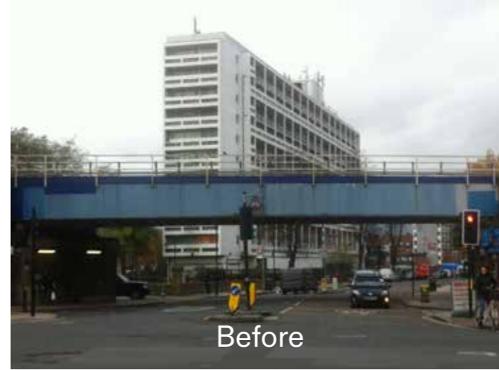
COMPLETED: Loughborough Road Bridge, "Mama Africa"
