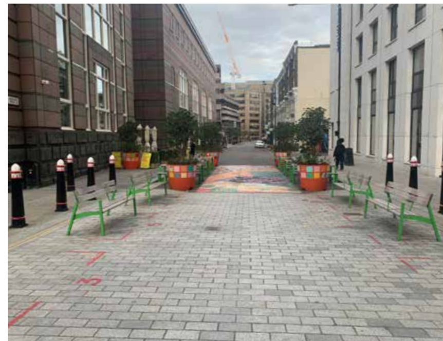
The existing raised surface at the southern part of Middlesex Street south will be retained as a turning space for vehicles.
