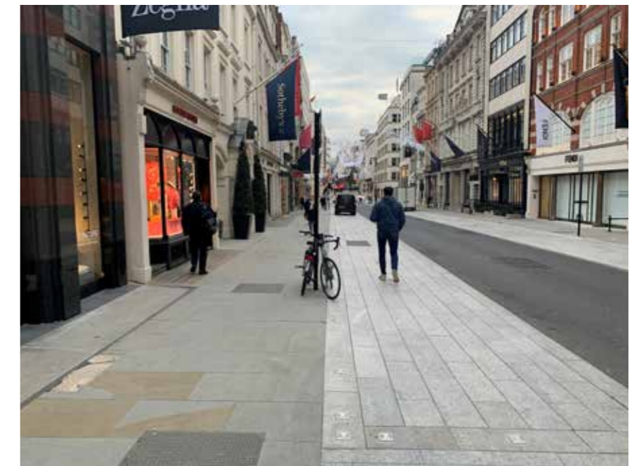
Example of recessed parking/loading facilities, New Bond Street.
