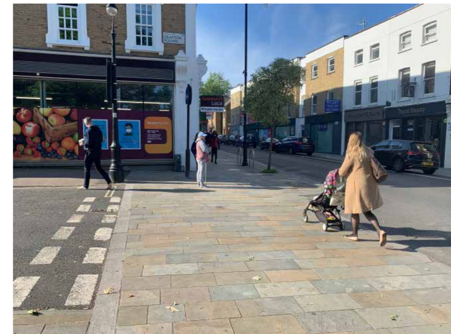
Continuous footway treatment maintains pedestrian priority at junction (Grafton Square).
