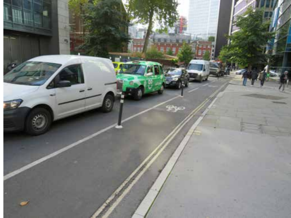
Protected cycle track on St. Botolph Street
