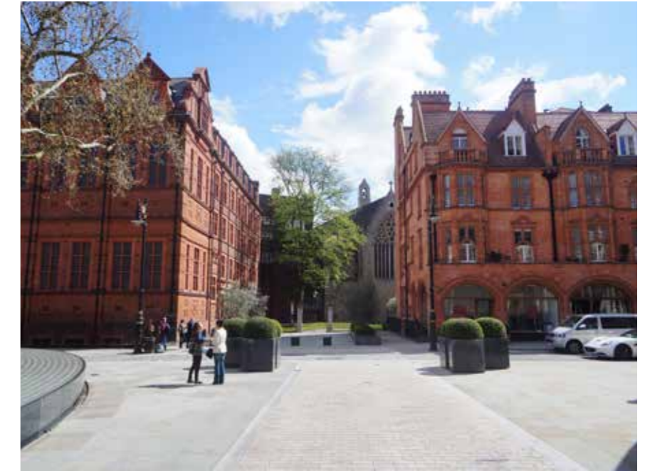
Pedestrian desire lines embedded across carriageway (Mount Street)
