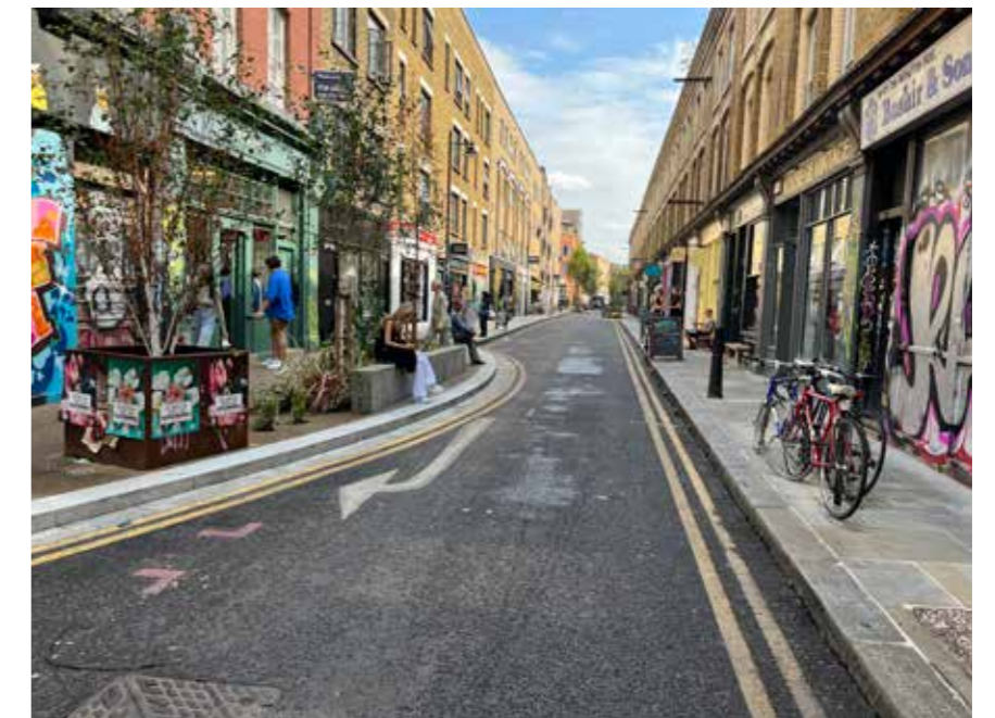
A build-out widens the footway, slows down vehicles and cycles and creates a small public realm with seating and planting (Cheshire Street)
