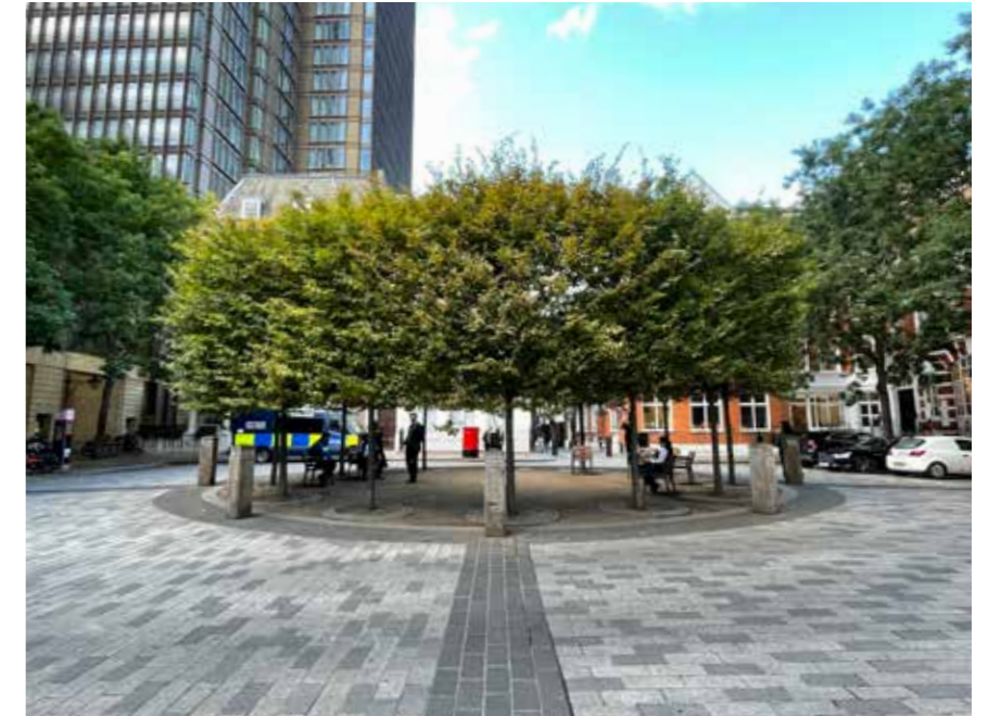
The carriageway in Devonshire Square has been raised to footway level and repaved to create a sense of square across the space.
