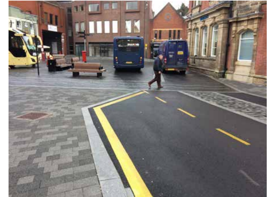
A loading and unloading bay design employed the concept of shared space and was paved with high-quality natural stone (Exchange Square, Kidderminster)
