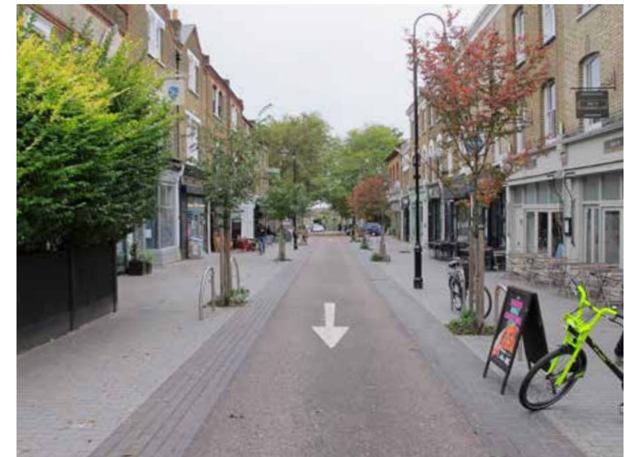
Orford Road has been redesigned with a single level surface approach with an asphalt strip on the middle of the street.
